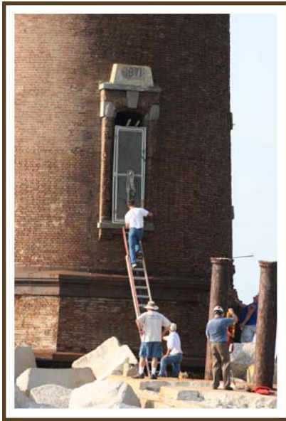
Lower window on north side of lighthouse used to access tower
