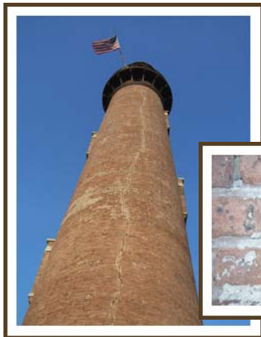
External Vertical Cracking on East Side of Lighthouse
